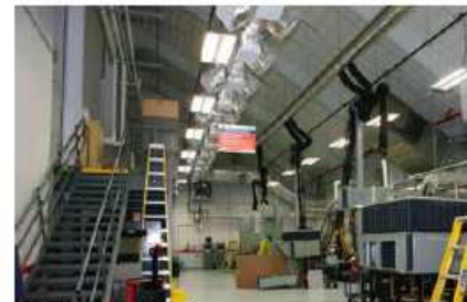
Gas Furnace Testing
